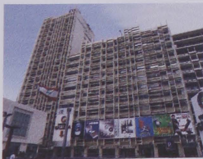
3- South Façade View
