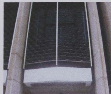
4- Closer View of the Façade
