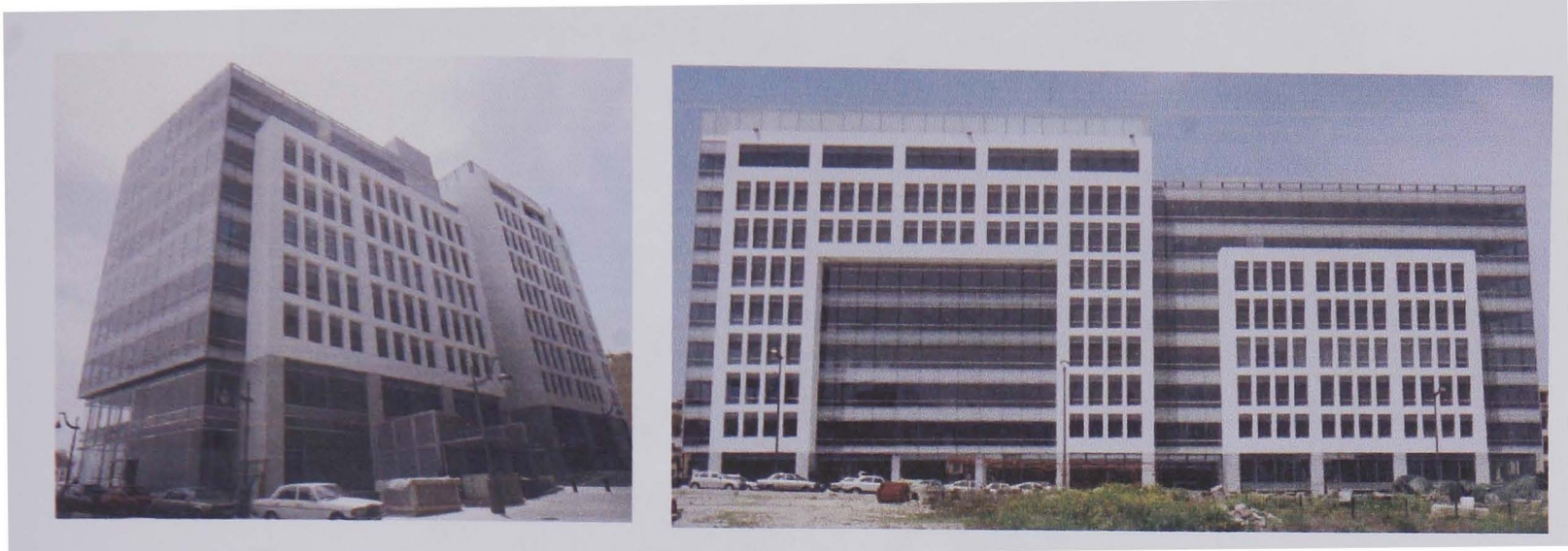
Figure 7.74. External views of El-Nahar office building (B35), D.O.C. 2002.
