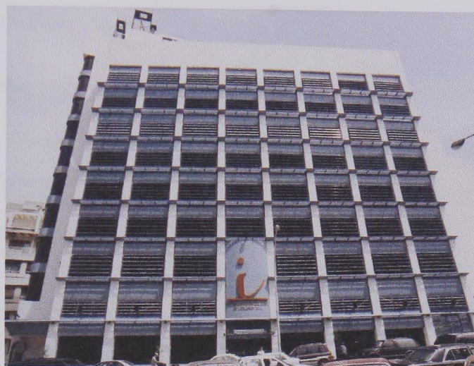
Figure 7.63. View of the renovated south façade of B30.
