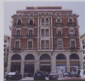
3- North Elevation View
