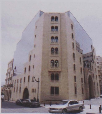
Figure 7.66. The M.P.s Office building, D.O.C. 1994.
