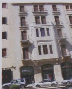
1- South Façade View
