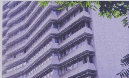
4- Closer View of the South Elevation
