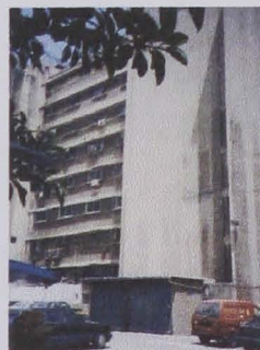
4- South Façade View
