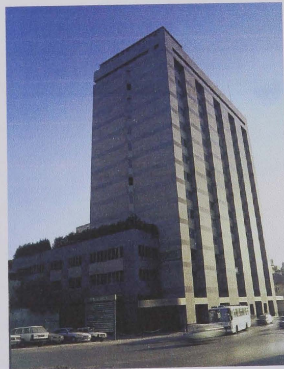
Figure 7.61. El-Ghazal Tower (B29), D.O.C. 1983.
