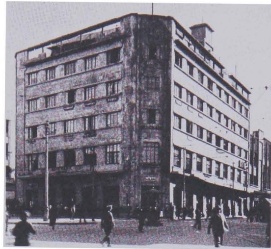
Figure 7.28. 'Ibrahim Sursok' Building (B06), D.O.C. 1935 (Arbid, 2002).
