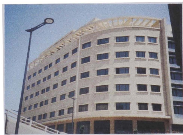
Figure 7.36. 'Riad Solh 1374' Building (B11), D.O.C. 1956.
