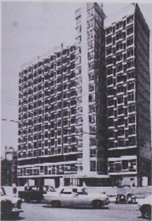
Figure 7.50. Electricity of Lebanon Headquarters (B21). D.O.C. 1965 (Tabet, 1998).
