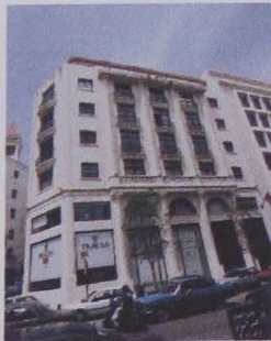
3- East Elevation View
