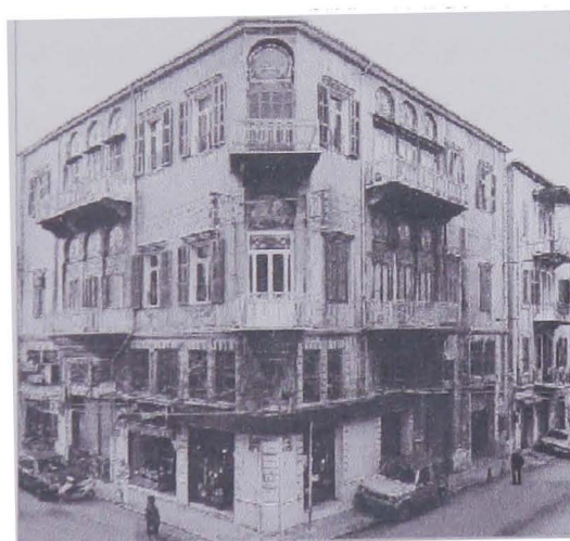
Figure 7.18. Barakat building (1923): the use of stucco finishing and horseshoe arch (Arbid, 2002).
