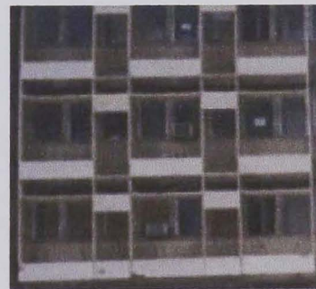
2- Closer View of the South Façade
