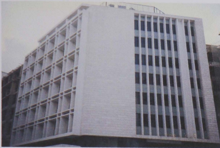
Figure 7.46. 'Riad Solh 1216' building (B17), D.O.C 1959.
