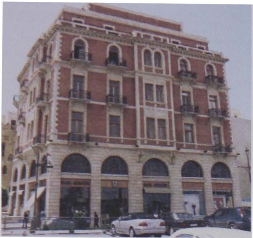
Figure 7.27. 'Fosh 1153' Building (B05), D.O.C. 1932.
