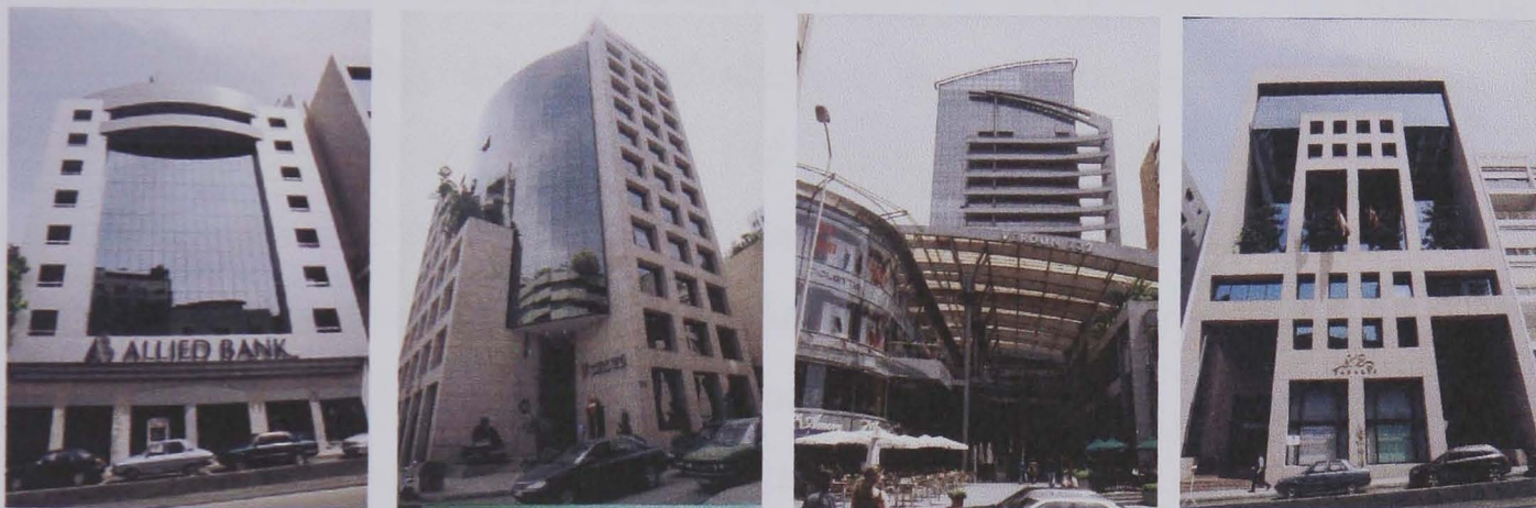
Figure 7.68. Examples of office buildings constructed during the last 5 years, in Beirut.
