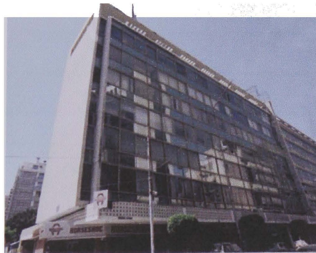
Figure 7.40. The Horseshoe Building (B16), D.O.C. 1957.
