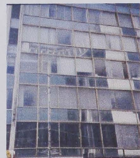
5- Closer View of North Façade
