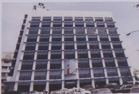
3- Renovated South Façade
