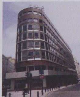
3- South East Façades View
