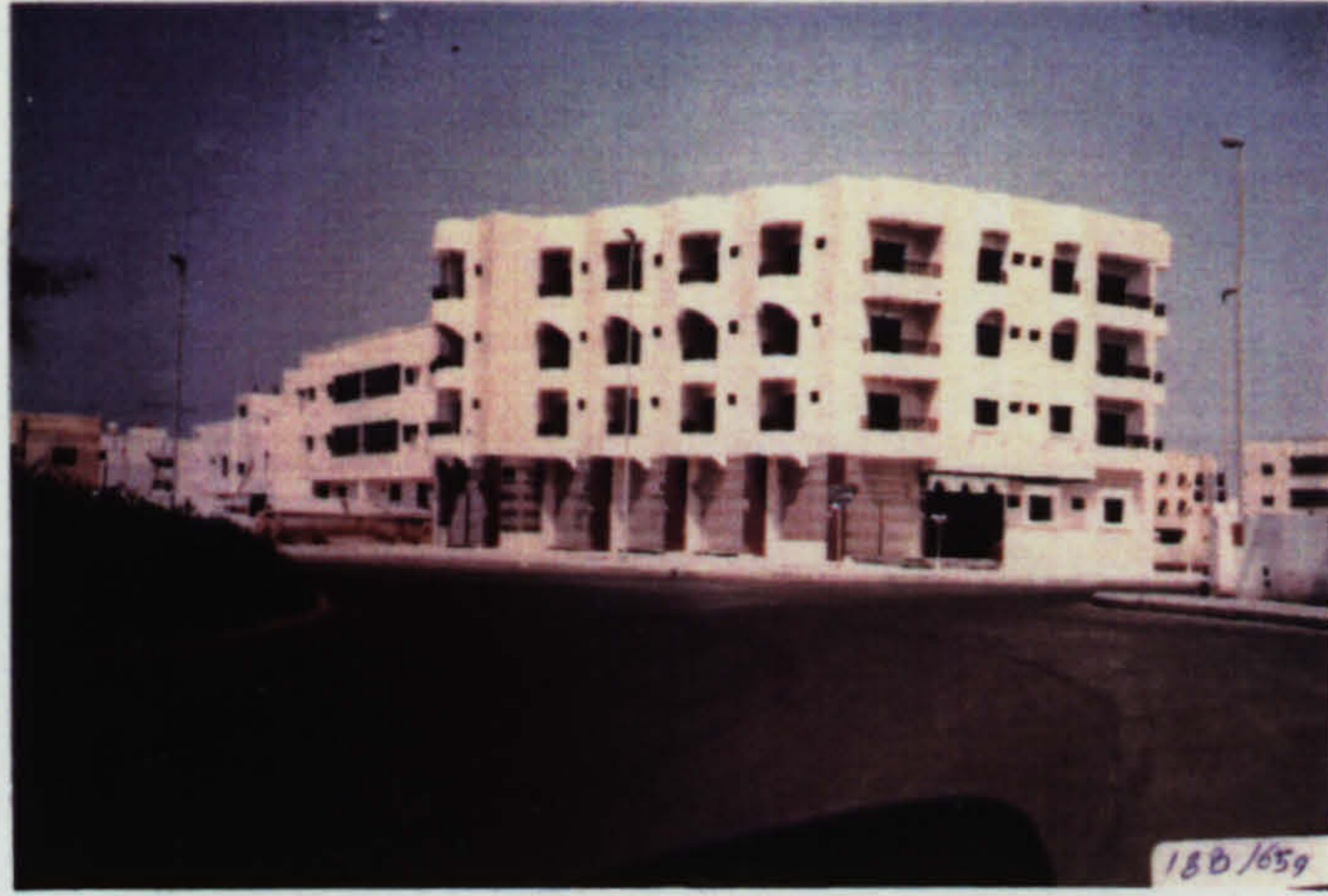
PHOTO 7.13 : View of building No.2
