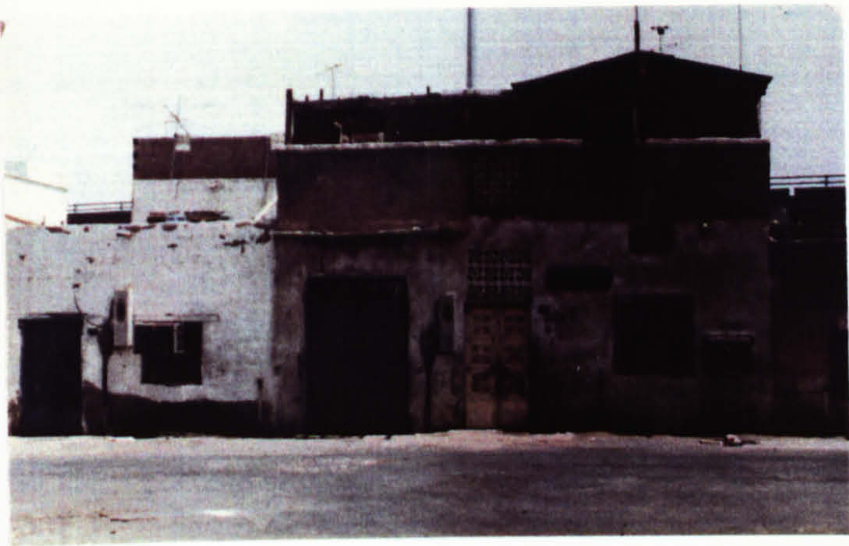
PHOTO 6.10 : Shows sandakah on the roof of Al Bayt Al Shabi
