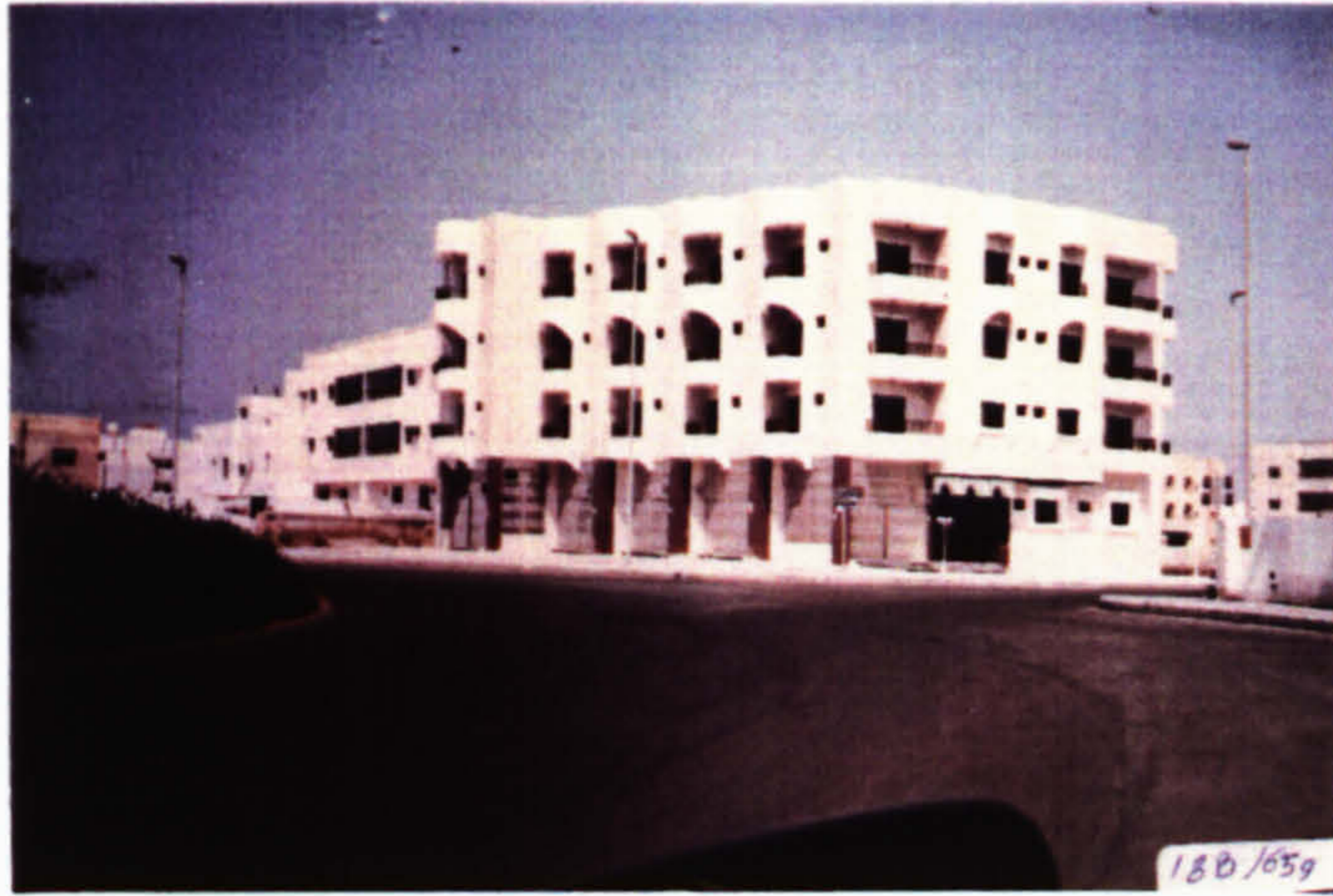
PHOTO 7.13 : View of building No.2
