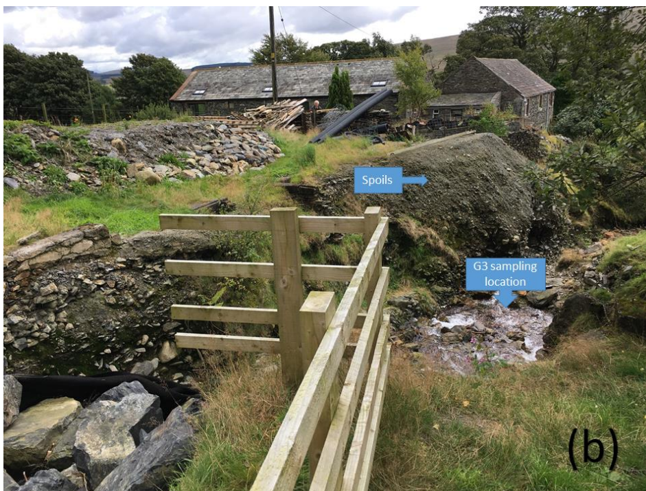
Figure 5.6: Location of mine spoil: (a) close to the bottom of the dam (b) besides G3 sampling location (photos taken on 14/09/2017)
