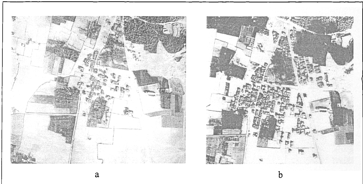
Fig.8.10: Growth of the post-oil neighbourhoods. a) Aththulaithiyyah Neighbourhood in 1960 (scattered houses with predetermined streets and land size and shape). b) Aththulaithiyyah neighbourhood in 1967 (the fereej system had been established and the density of the area had increased). Notice how the green areas around the city had been abandoned to be used for residential purposes. Source: Based on Aerial photographs (1960 and 1967), Aramco.
