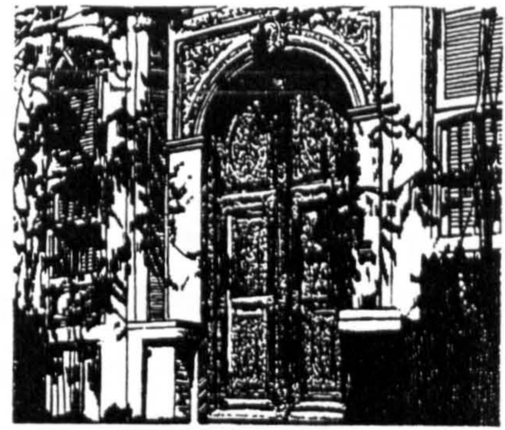
Figure 1.3 – A decorated gate of one of the traditional houses in Jeddah. Source: Pesce, 1977: 119.
