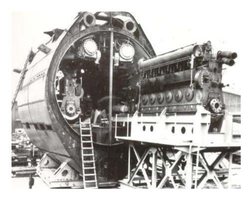
Figure 2.2 - U-Boat construction in WWII, showing advanced blocks being used (source: forum.axisindustry.com)
