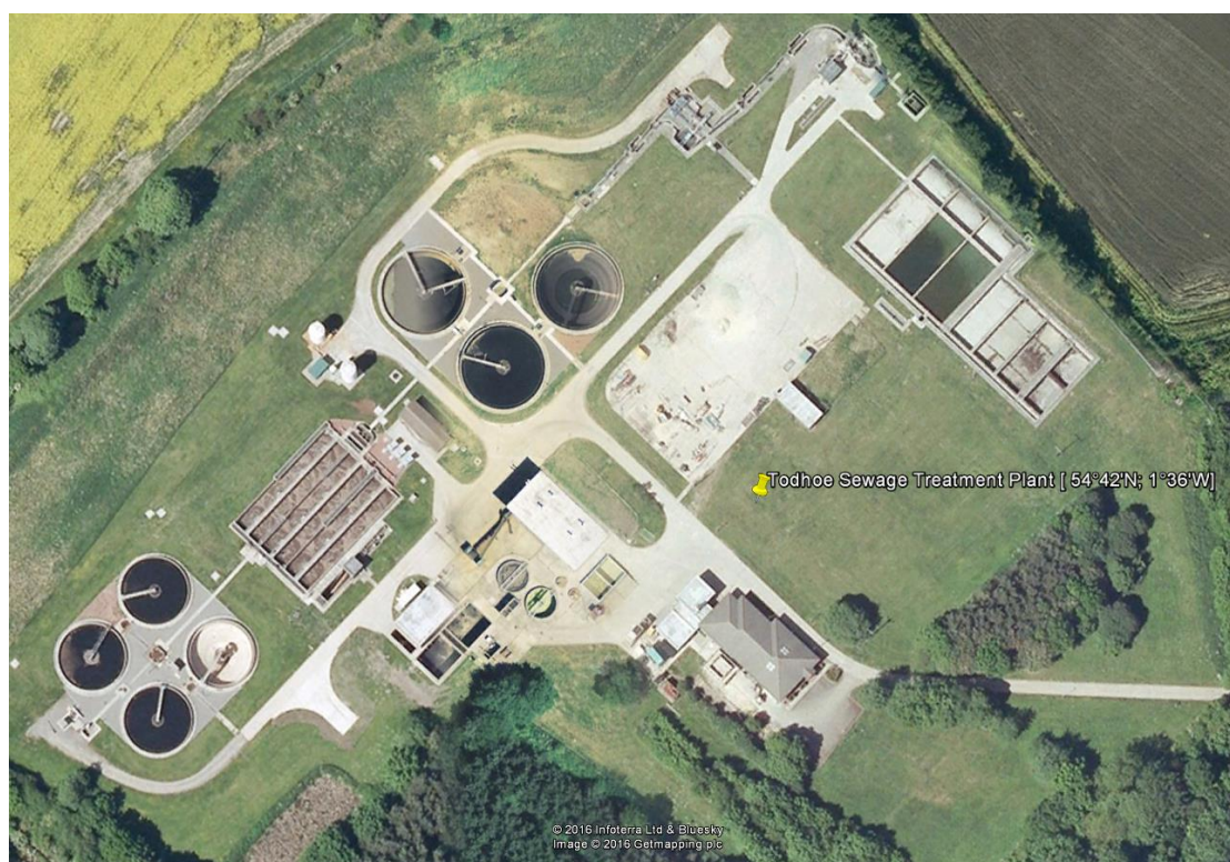
Figure 3.4: Satellite image of Tudhoe Sewage Treatment Plant, UK. [Courtesy of: Imagery ©2016 Getmapping plc, Infoterra Ltd & Bluesky, Map data ©2016 Google]
