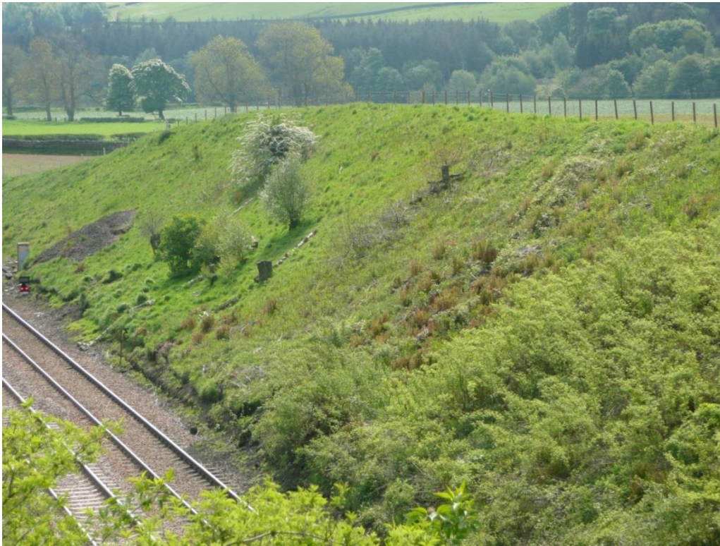
Figure 3.4: A cutting earthwork approximately 2.6 km east of Haltwhistle. The adjoining fields indicate the heterogeneous nature of the vegetation cover in the study area.
