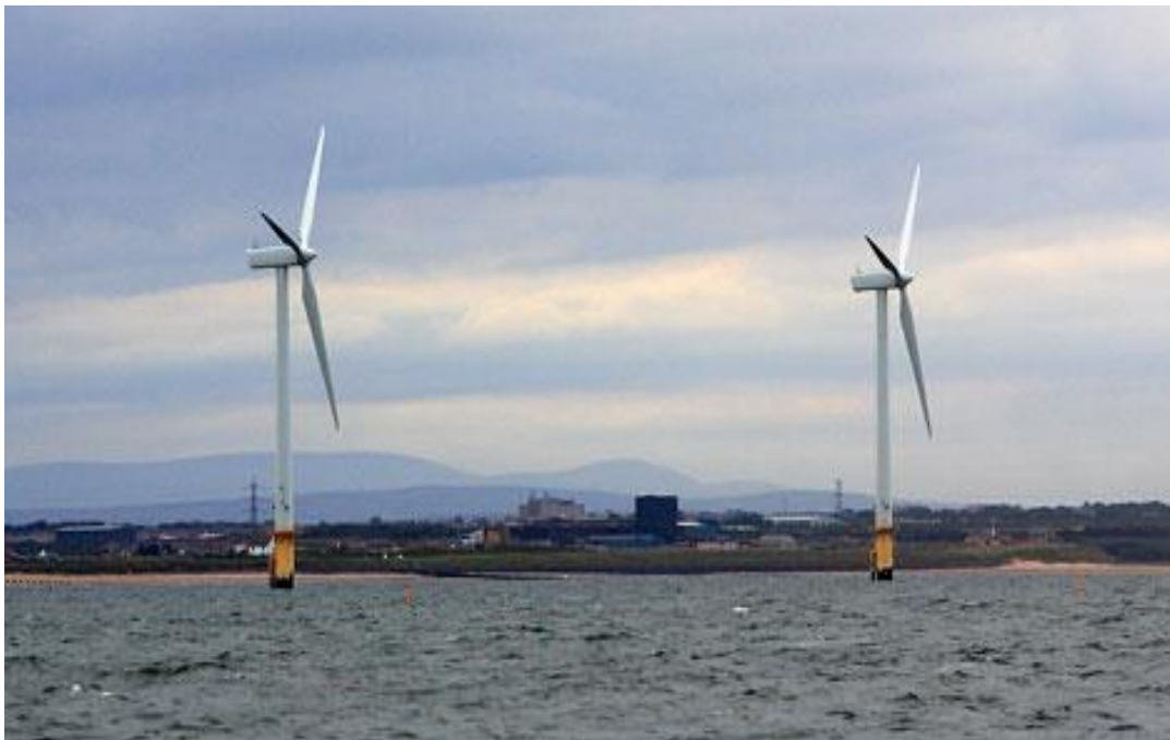
Figure 4.2 Blyth Offshore Wind Farm
