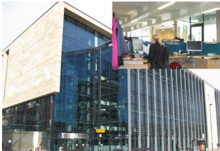
Figure 37 King's Gate's glazed front provides ample daylight in office areas, which are complemented with fluorescent artificial lighting.
