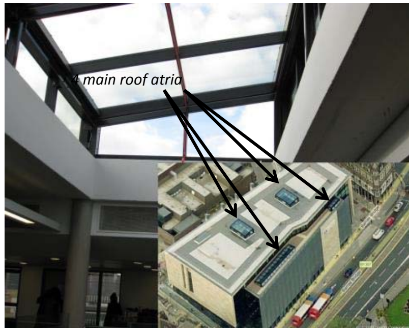
Figure 10 Roof-top atria intended to admit daylight and facilitate natural ventilation
