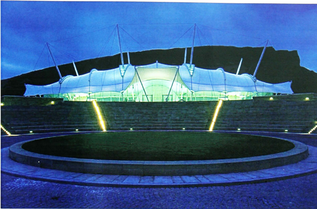
Figure 1-4. Dynamic Earth Centre, Edinburgh, UK (Arup)
