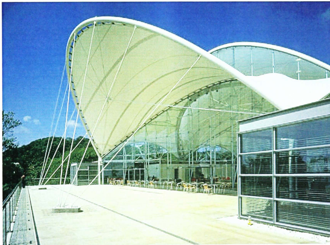
Figure 1-1. Saga headquarters, UK (Arup)
