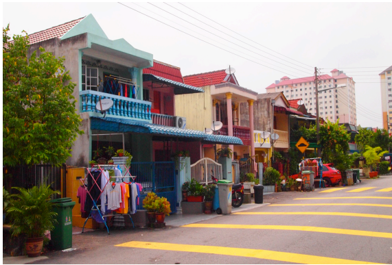
Figure 52 Low-cost two-storey houses were renovated without conforming to regulations (Picture taken by author)
