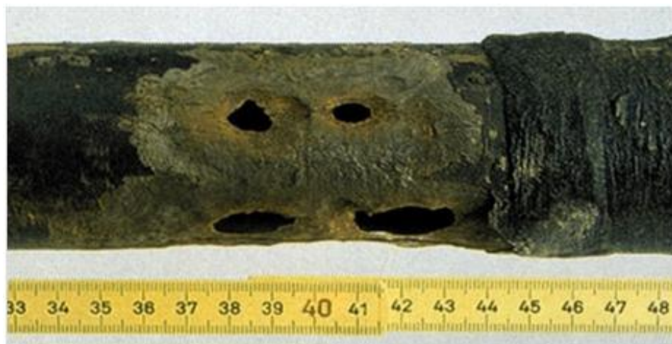
Fig.2.6: Failure of a gas supply pipe due to an earth leakage current
