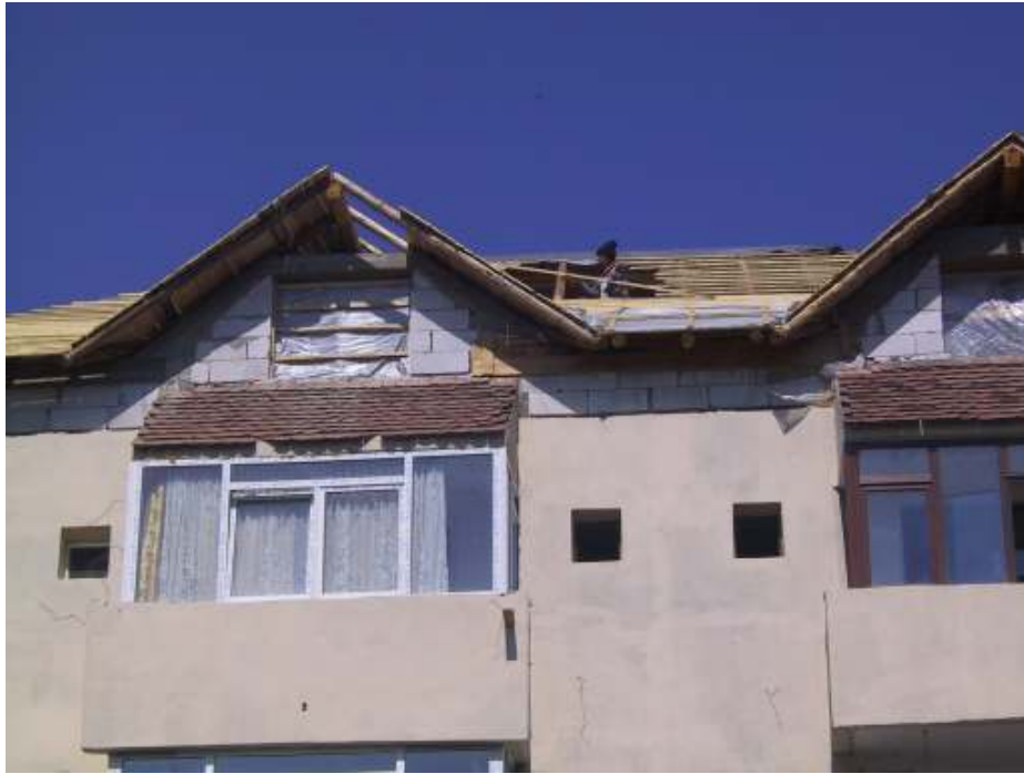
Figure 8.11: Constructing a new flat on the top of the building
