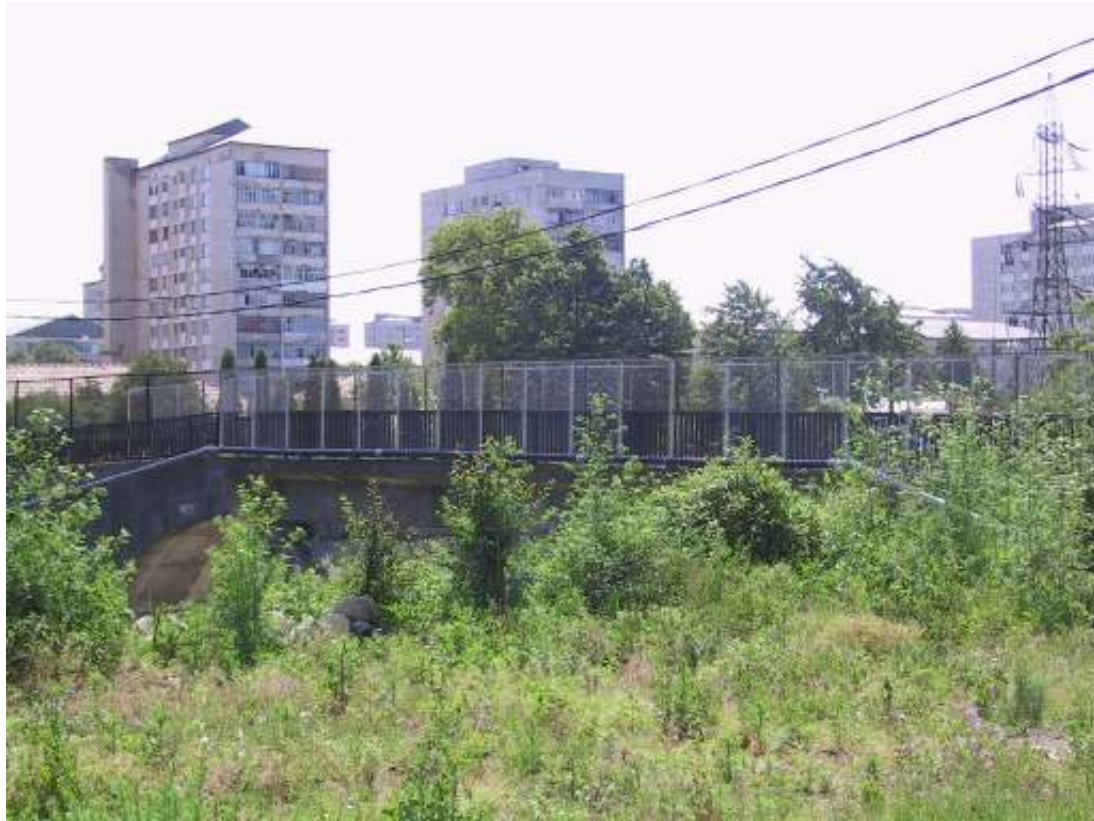
Figure 8.10: Blocks of flats used for the re-allocation of the Roma Community in the area of Darmanesti in Neamt
