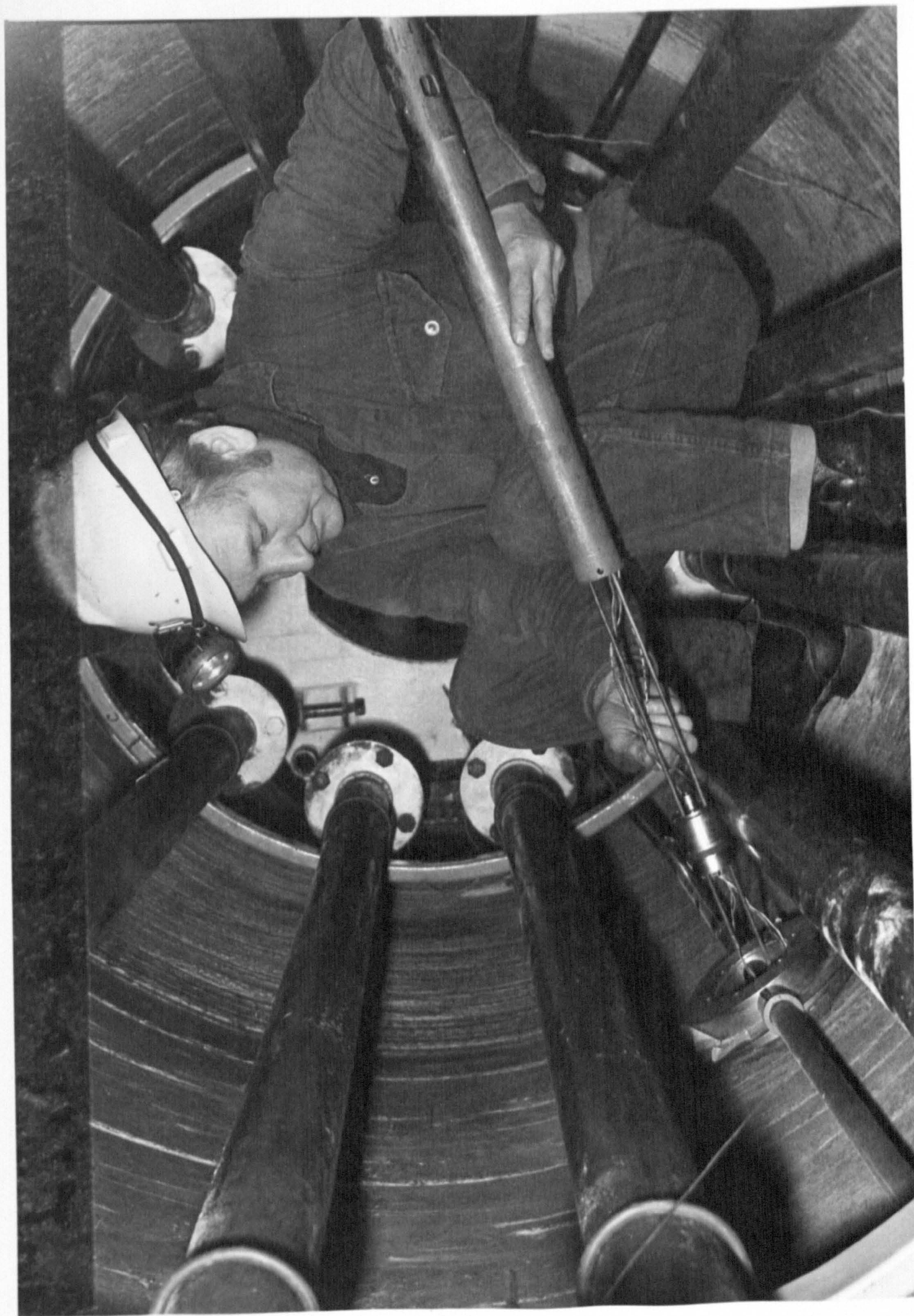
FIG. 30 INSERTION OF ANCHOR NO. 3
